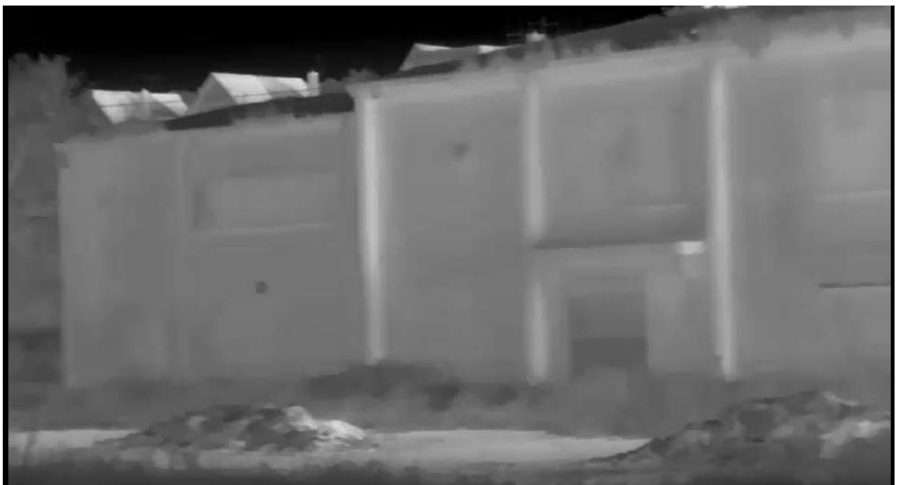
Plate 6: Side of sports hall surveyed by Thermal Imagery during Dawn Survey 25/8/2021.
