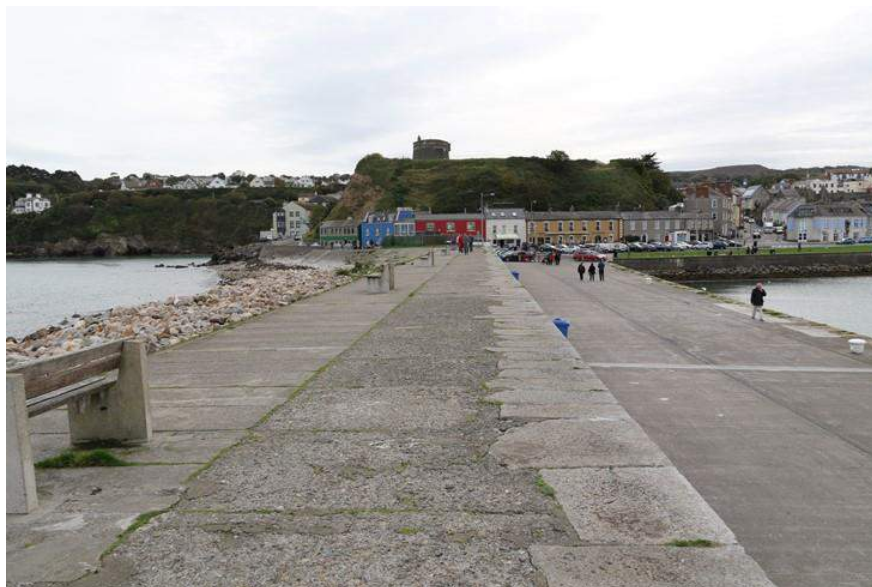
Plate 13: View of Martello tower from the East Pier
