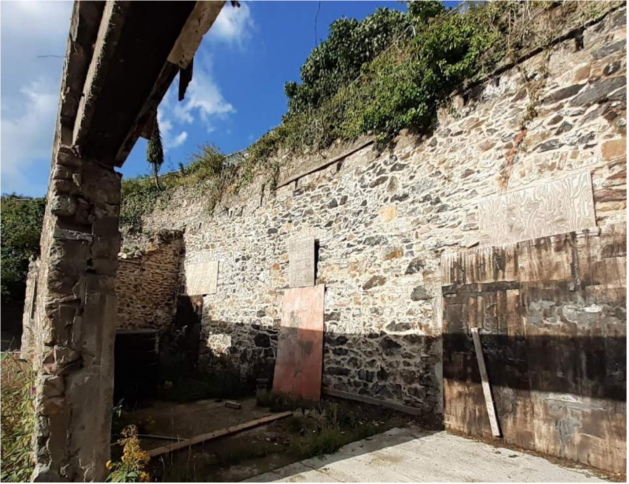
Plate 3: Vaults of former Baily Hotel, Howth, Co. Dublin.
