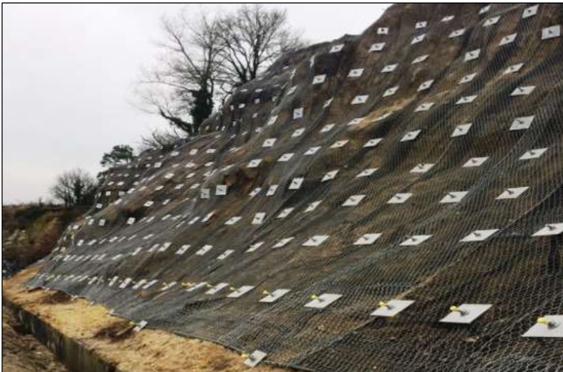
Figure 9.3 Soil Nailing Example, prior to vegetation re-growth
